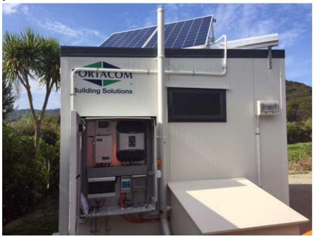
The Quarry system is a small off grid system that we designed for Ron Gorter at Fulton Hogan. The entire system – modules, inverter and batteries - are designed to be easily "de-mountable" and thus allow the Portacom to be relocated to its next site when necessary.
